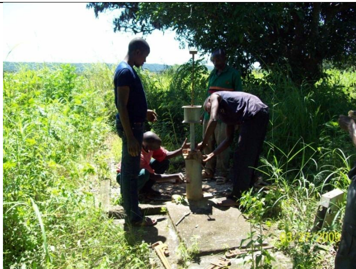
The Pump Repair crew quickly determines what repairs are needed.
